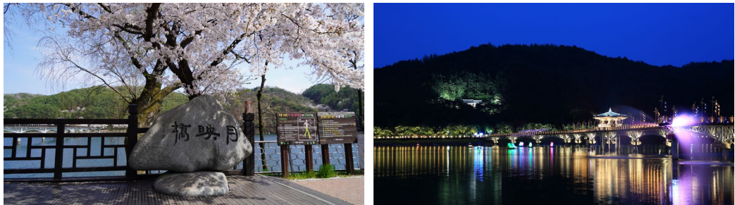
Wolyeong Bridge in spring and the bridge's night view
